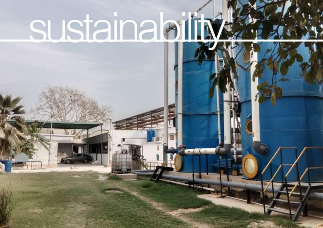
To ensure that we meet our commitments, we have our own Self-Generation Prime Power Plant to supply uninterrupted power and to further reduce emissions we installed waste heat recovery boilers to supply saturated steam to the processing unit.
